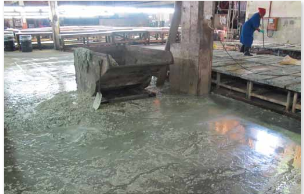
General housekeeping practice at this facility
