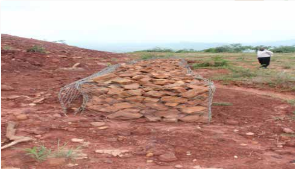
Picture 3: Hilltop 01 with a gabion placed thereon by the offenders in an attempt to prevent or minimise the soil erosion.
