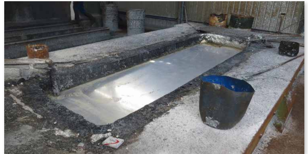
Picture: Hot Dip Galvanising
