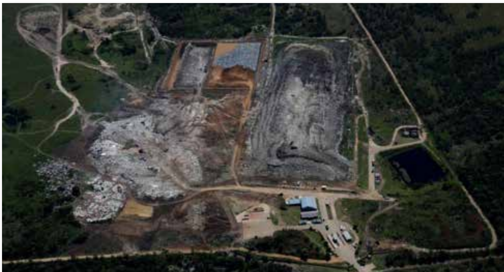
Picture: Uncovered, uncontained, uncontrolled.
